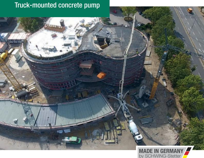
Vertical reach 50.10 m Concrete output max. 162 m $^3$ /h Pressure on concrete max. 85 bar Tare weight < 40 t
